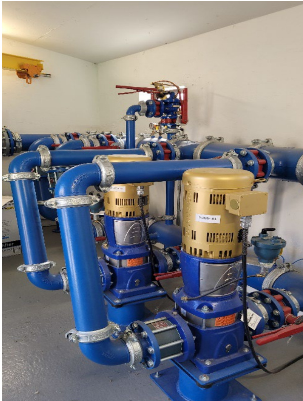
Photo 5-4: Strahorn Booster Station
