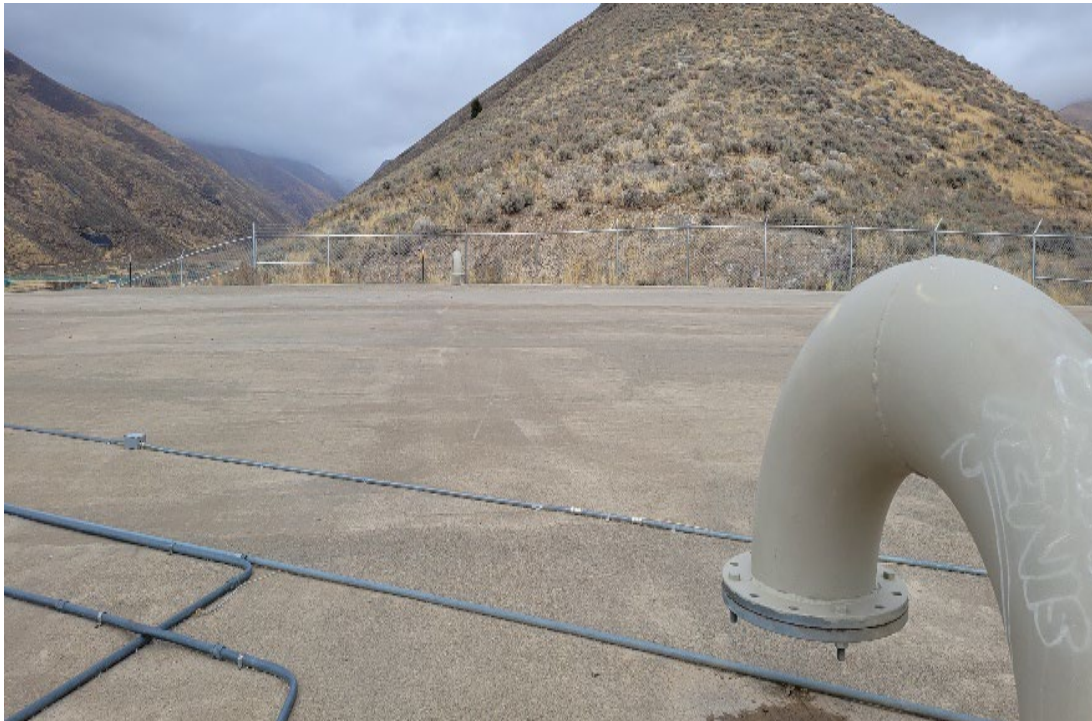
Photo 5-3: Top of Reservoir
