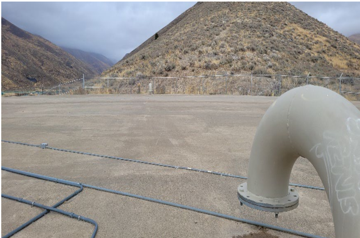
Photo 5-3: Top of Reservoir
