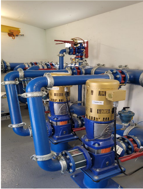
Photo 5-4: Strahorn Booster Station
