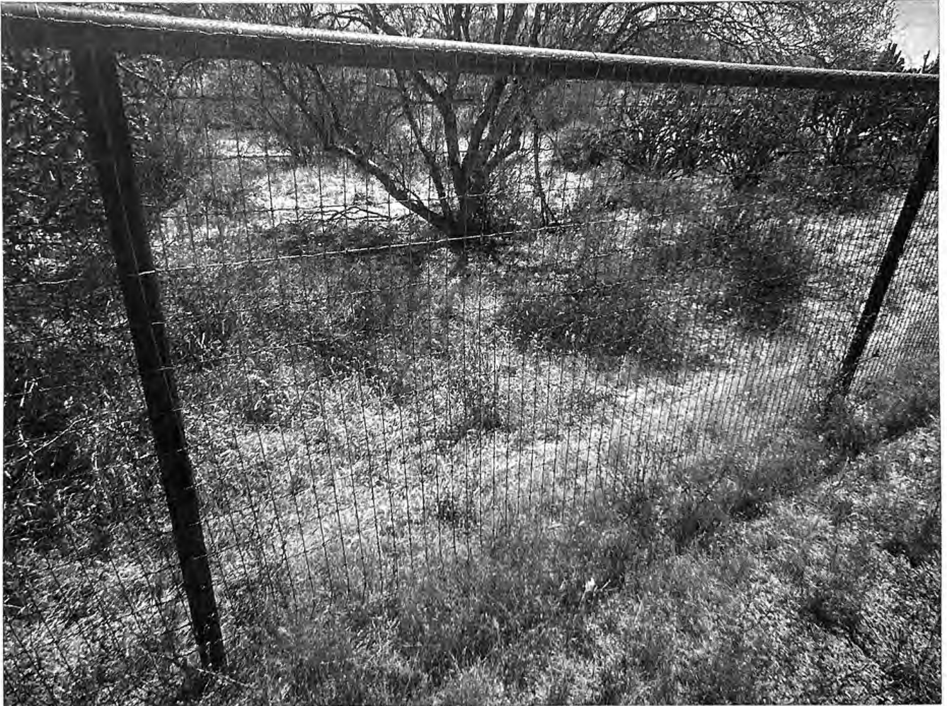
Applicant-provided fence style reference (single-rail pipe top with welded-wire critter mesh; corner pipe post).
